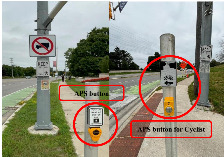
Figure 4.3: APS at an intersection. (Source: Original Photograph by Samuel Olugbade 2024, August 8, 2024).
