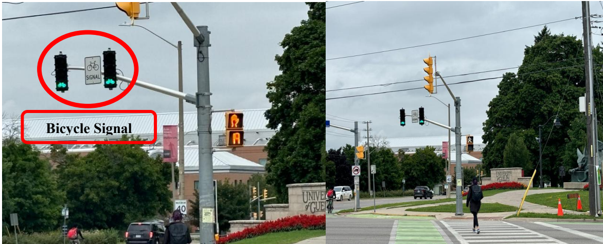
Figure 4.2: Implementation of the Bicycle Head Signals and Bicycle Signal Head on Green Signal. (Source: Original Photograph by Samuel Olugbade 2024, August 8, 2024).
