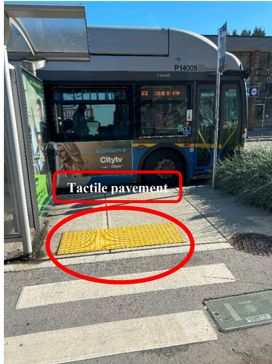
Figure 2.7: The Tactile pavement. (Source: Original Photograph by Samuel Olugbade 2024, August 8, 2024).
