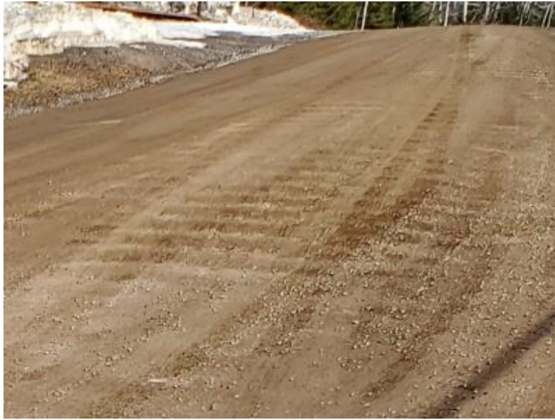
Figure 5: Washboarding (corrugation) of an unpaved road surface
