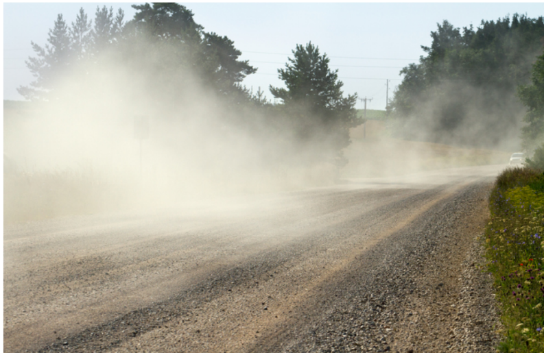
Figure 9: Dust on an unpaved road surface (From Oransi 2021)
