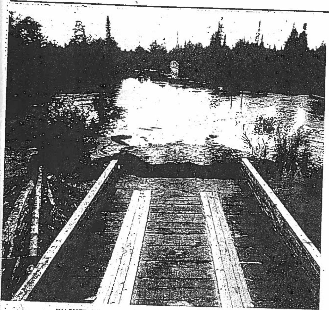
WASHED OUT ROAD LEADING TO RESERVE 22A2 WEDNESDAY
