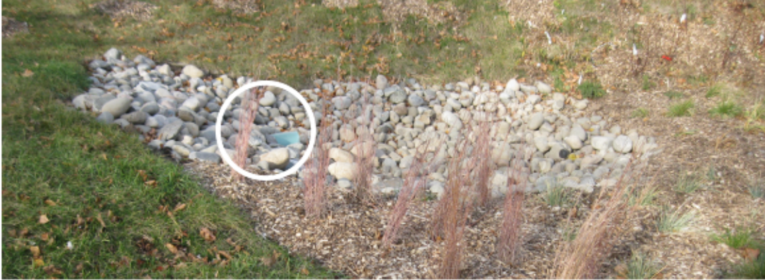
Figure 12. West LID entrance and pre-treatment and feeder pipe (white circle) (McVicar Creek LID)
