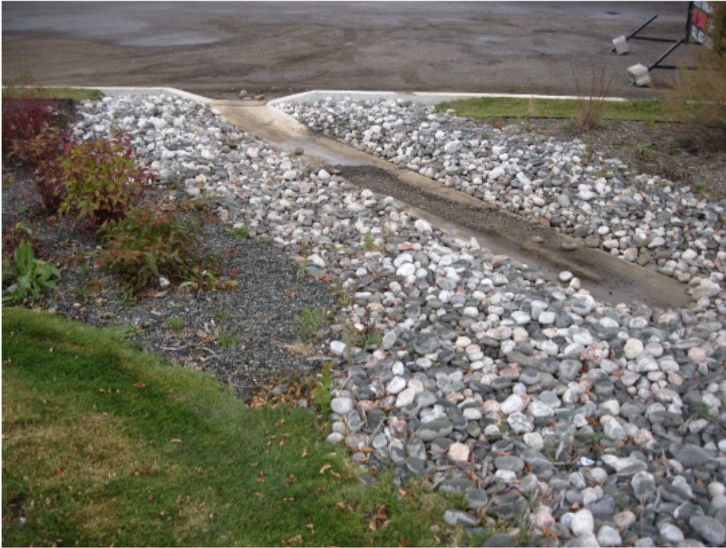
Figure 8. D&R Sporting goods LID entrance and pre-treatment
