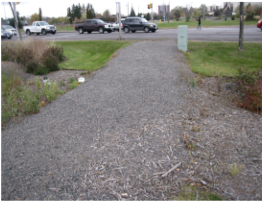
Figure 10. Storm drain (D&R LID)
