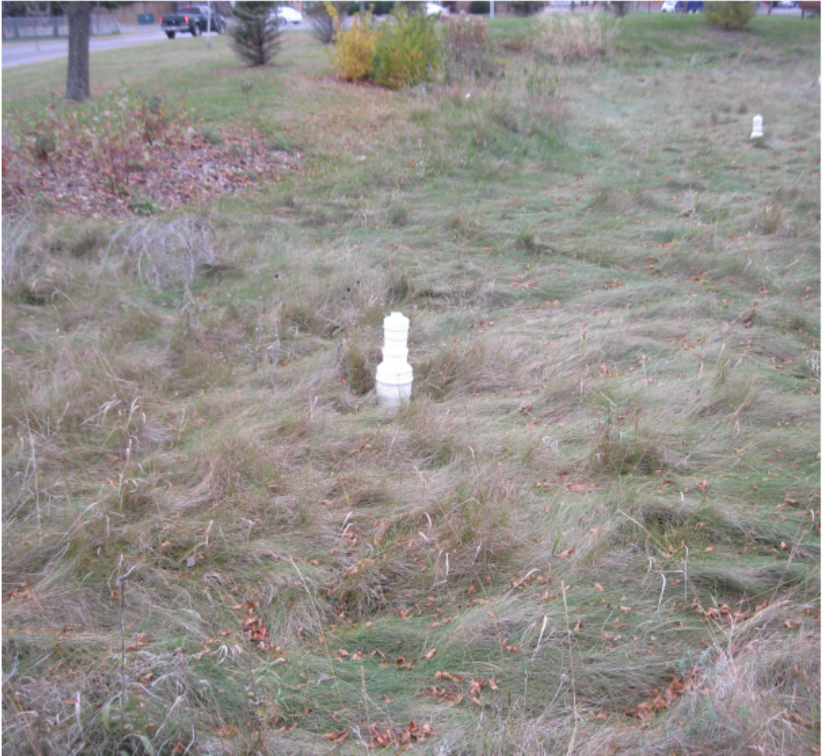
Figure 7. Drain pipe observation stations (Beverley Street LID)
