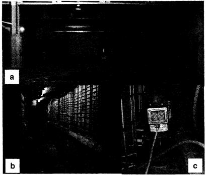
Figure 7 - Effluent storage for the flow-through experiments: a - cold room (outside) on  $3^{rd}$  floor of AbitibiBowater newsmill. b - cold room (inside) and 1050L storage tanks. c - agitator motor used for stirring and dechlorination
