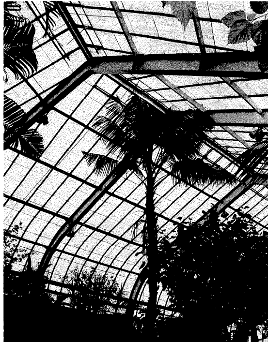
Figure 5.1. A photograph of the glass roof boundary taken inside the Conservatory.
