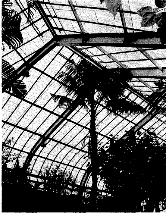
Figure A.2. A photograph of the glass roof boundary taken inside the Conservatory.
